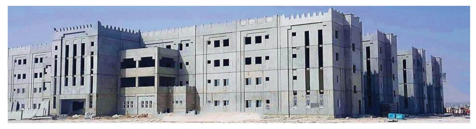
Precast concrete is a construction product that is produced by casting concrete in a reusable mold. It is cured in a controlled environment, transported to site and lifted into place. Precast concrete is a highly versatile product available in vast range of different sizes, functions and finishes.
